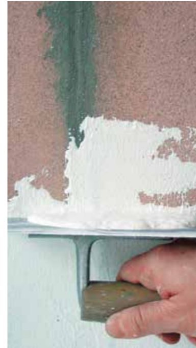
(4) Total leveling treatment with a coat of rialto raselast
