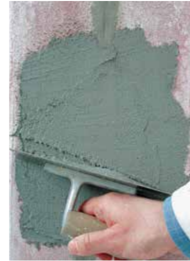
(4) Total leveling treatment with a coat of rialto intonal or mixture based on rialto matonal
