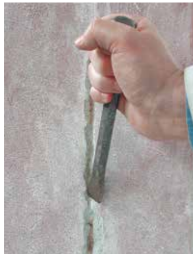
(1) Expanding the crack
