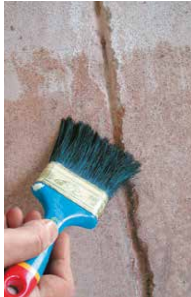
(2) Application of rialto primer (interior walls) or rialto stabilizer (exterior walls)
