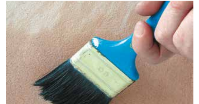
(2) Application of rialto primer (interior walls) or rialto stabilizer (exterior walls)
