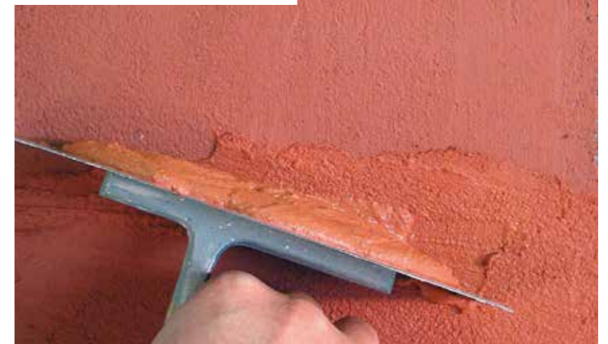
(7) Application of the selected rialto thick coating
