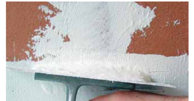
(3) Leveling with rialto raselast
